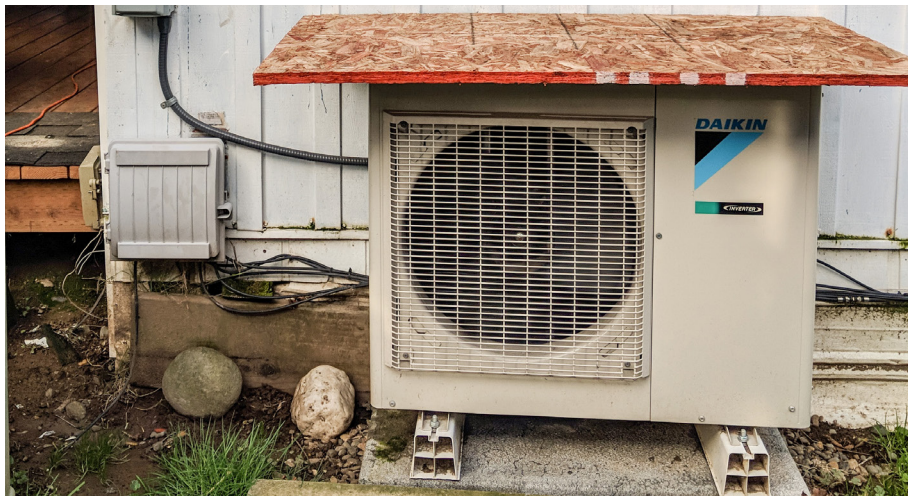
The exterior element of a ductless heat pump.
